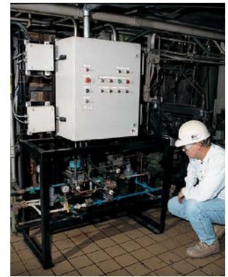
A standard valve rack with control panel is factory wired and tested to reduce installation time and cost. This valve rack can be conveniently located anywhere near the burner front.
