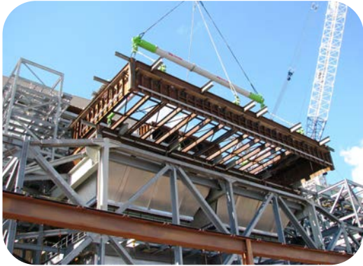
Modularization enhances quality and safety, and reduces schedule risk.
